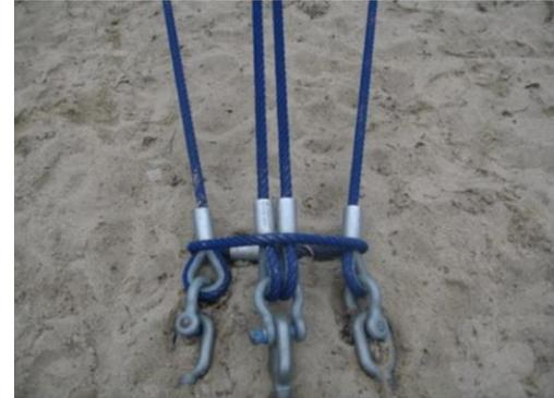
Huge spacenet structures are secured to the foundation with a system of three turnbuckles. Horizontal and vertical edge cables are fixed to individual turnbuckles, which then connect to individual steel anchors. This system ensures that each edge cable can be tensioned separately and increases structural safety by way of independent anchoring.
